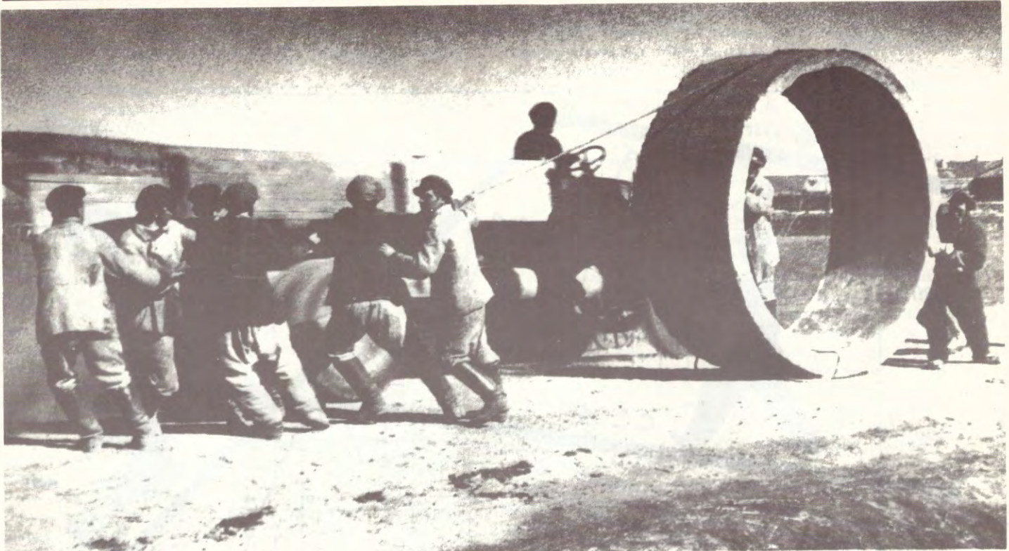
Magnitogorsk: a new metal plant being built during the First Five Year Plan.
